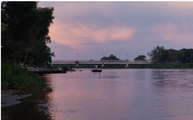
A raft crosses the Suchiate at dawn where people line up for passage on the bridge. Photo: Rene Soza
